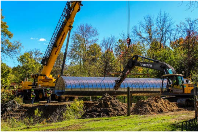
Verne Rd - Taymouth Twp Culvert Replacement
