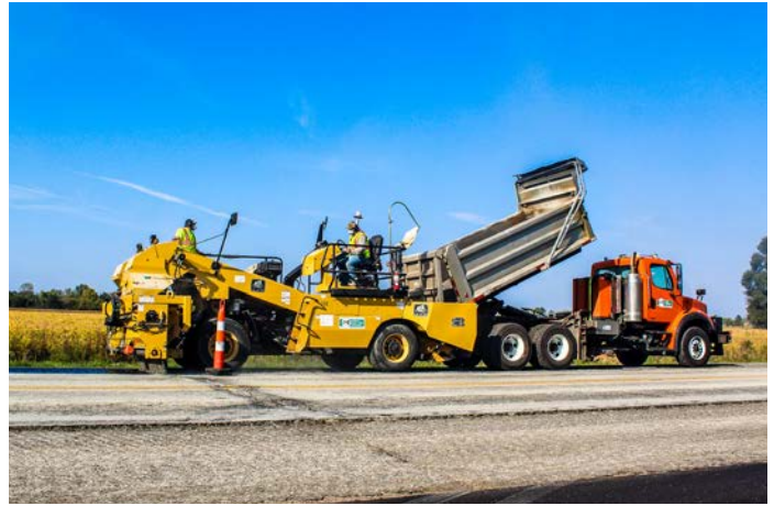
Dixie Hwy (Junction & Willard) Bridgeport / Birch Run Twps - Chip Seal
