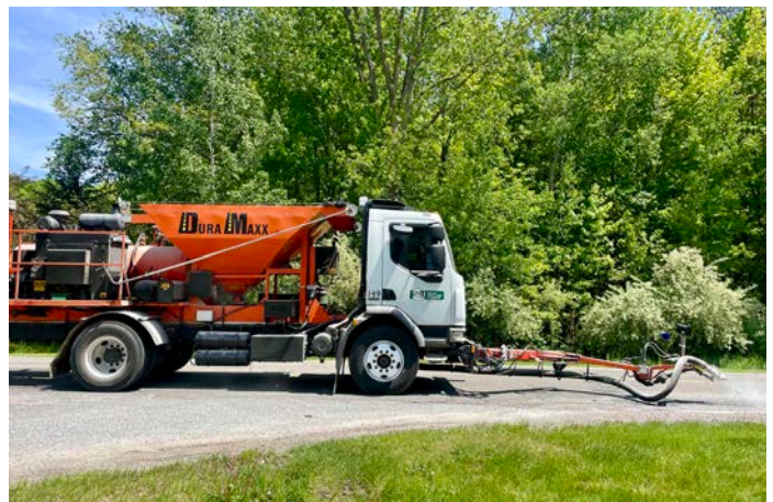
Countywide Road Patching
